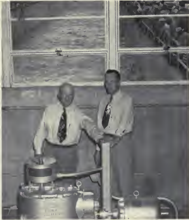
AT THE CONTROLS of the outlet works of Horsetooth Dam when water was released for the first time in July 1951 are the author, J. M. Dille (at left) and South Platte River District Manager J. H. Knights of the Bureau of Reclamation. Photo by N. T. Novill, Region 7 photographer.
